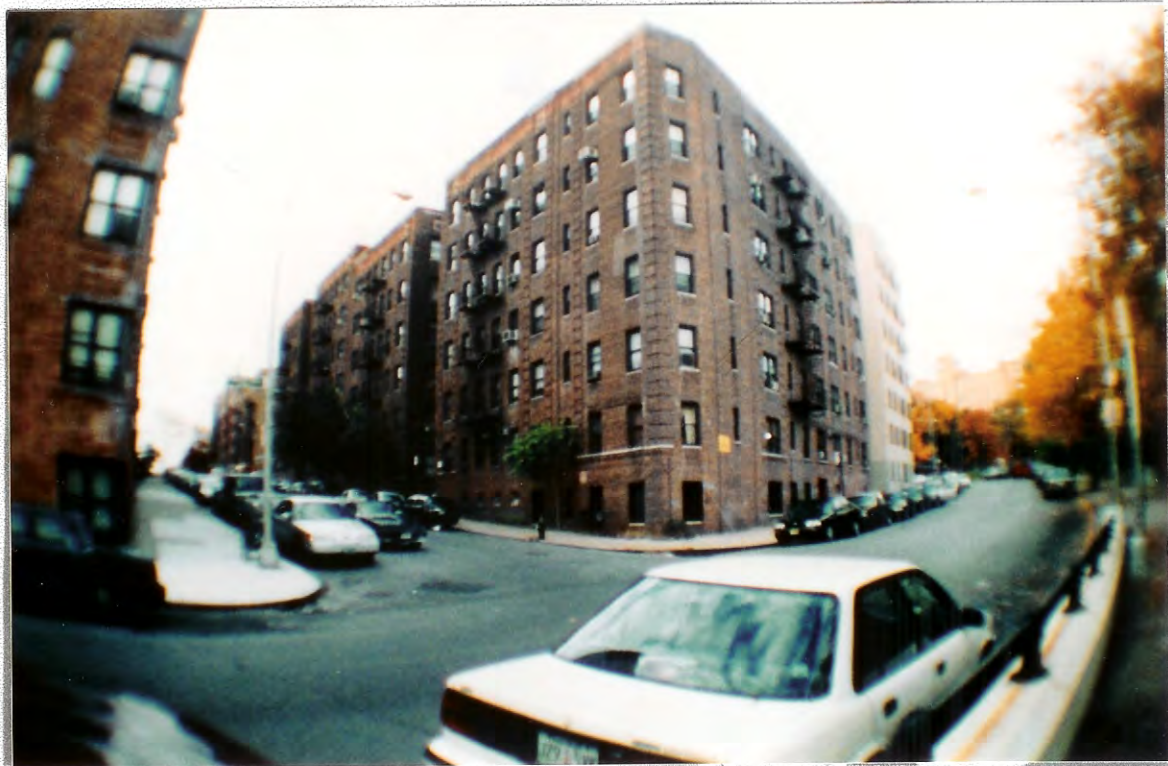
North West view. 485 West 187 Street, Apt. 1D.
